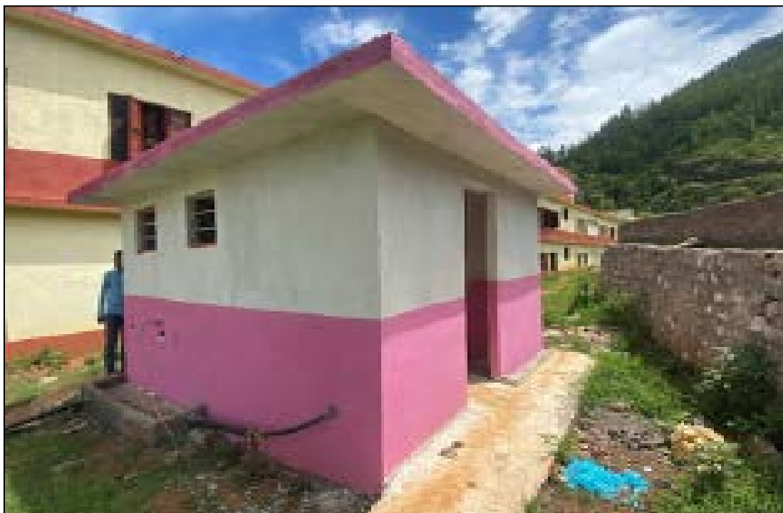
The toilet block at Shital Secondary School in Rukum, Western Nepal.
